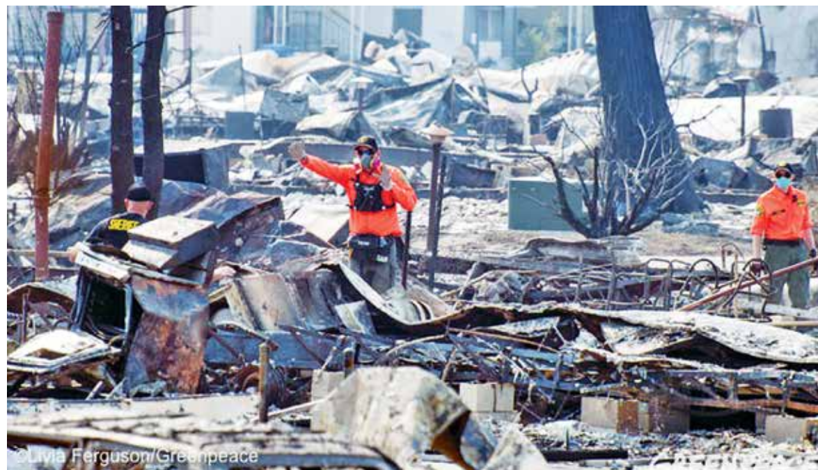
Fires destroyed thousands of buildings and homes in Sonoma County’s largest city, Santa Rosa. Burned to the ground was the greater part of a large working-class neighborhood, a mobile-home park, and three expensive hillside developments. PHOTO/LIVIA FERGUSON, GREENPEACE
