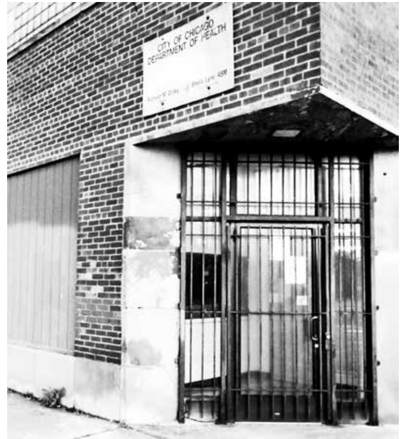
Boarded up mental health treatment center in Chicago.
