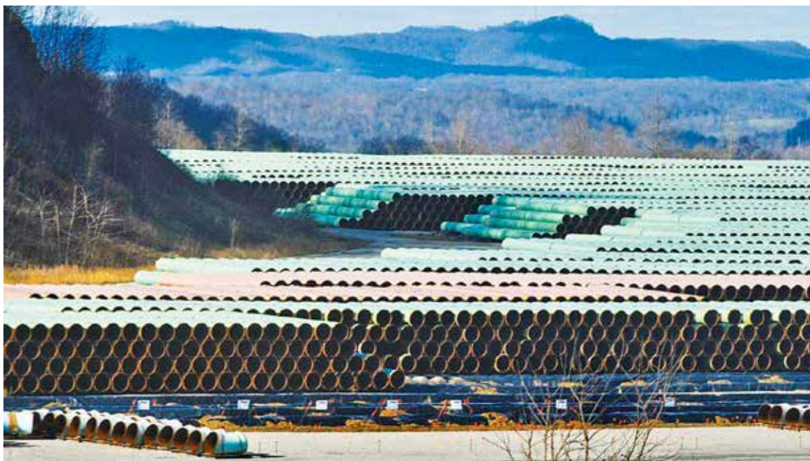
Pipeline construction staging area near Beckley, West Virginia. The Appalachian pipeline project will have devastating impacts on the scenic landscape of the Appalachian Trail, local drinking water, and the economy. Communities are resisting. PHOTO/T. PAIGE DALPORTO
