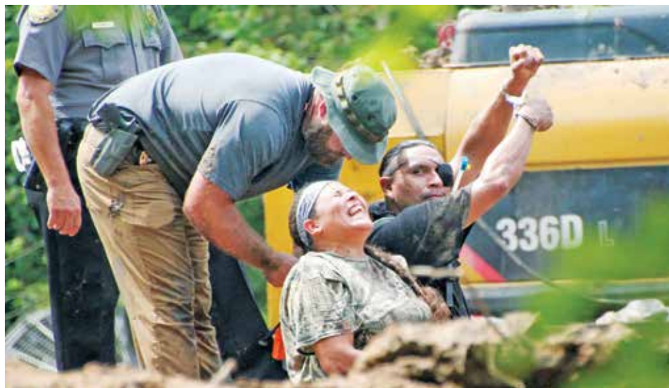
Water protectors are arrested at the site where Energy Transfer Partners is illegally constructing the Bayou Bridge Pipeline which threatens land, water and humanity.
