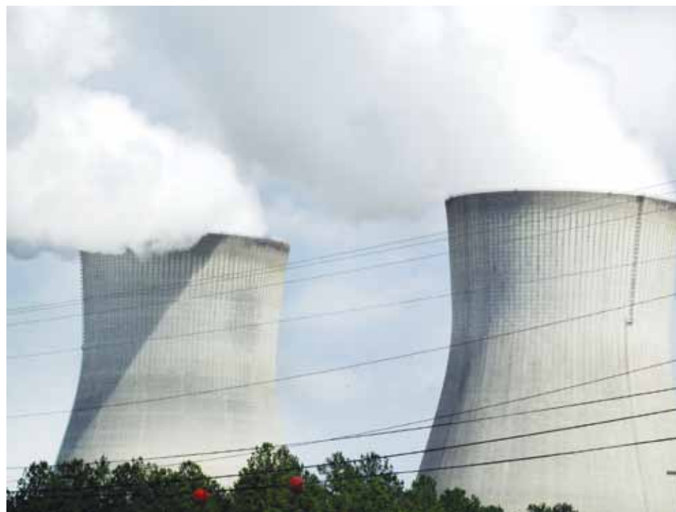
Cooling towers for nuclear power plants in Shell Bluff, Georgia.
