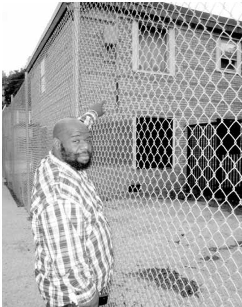
Former Cabrini Row House resident Henry Warfield points to windows improperly boarded up by the Chicago Housing Authority. The glass has been removed, allowing snow and rain to seep in and cause water damage, mold infestation and blight. Many residents say this was done purposely in order to force demolition. This translates into more contracts for private corporations.
