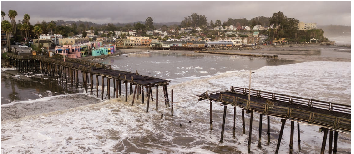
Powerful waves destroyed a large section of the wharf in Capitola, California during the atmospheric river storms.
